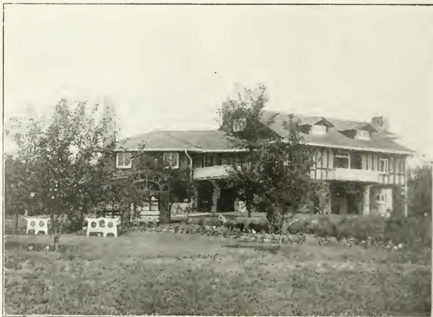
JAMES RYRIE'S RESIDENCE AT OAKVILLE
